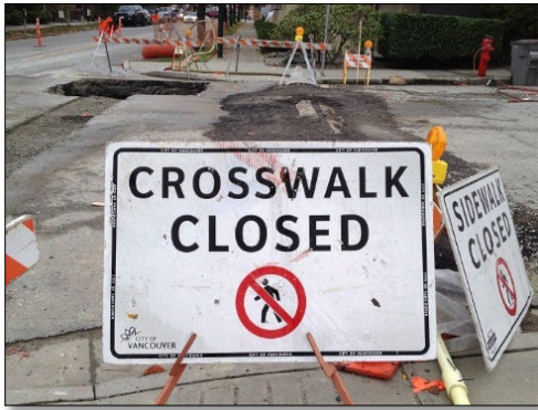
"Crosswalk closed" signs to be used at intersection or crossing. 900 x 600 mm.
