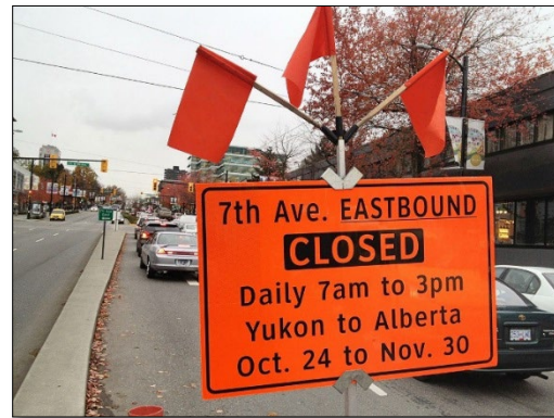
Example road closure advisory signs, with dates and times as appropriate. 900 x 600 mm or other sizes as appropriate.
