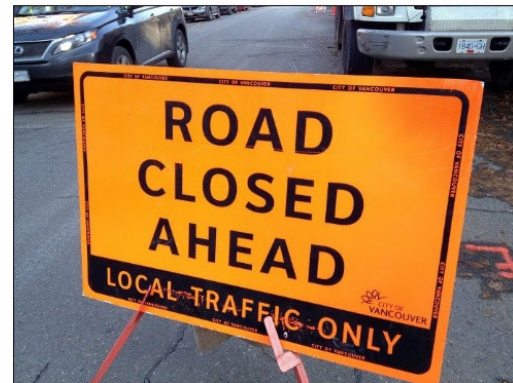
"Road closed ahead" sign to be used at intersection or decision point in advance of closure where motorists can detour around closure. 900 x 600 mm.
