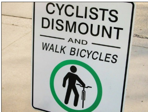
Example "cyclists dismount" signs to be used where cyclists are directed to use pedestrian facilities. Sizes as appropriate.
